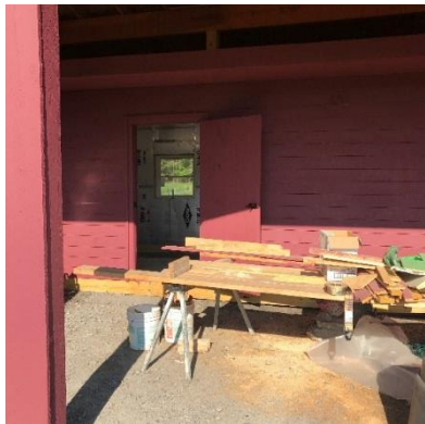
Construction on Deborah's Wool Room in the Tractor Shed
